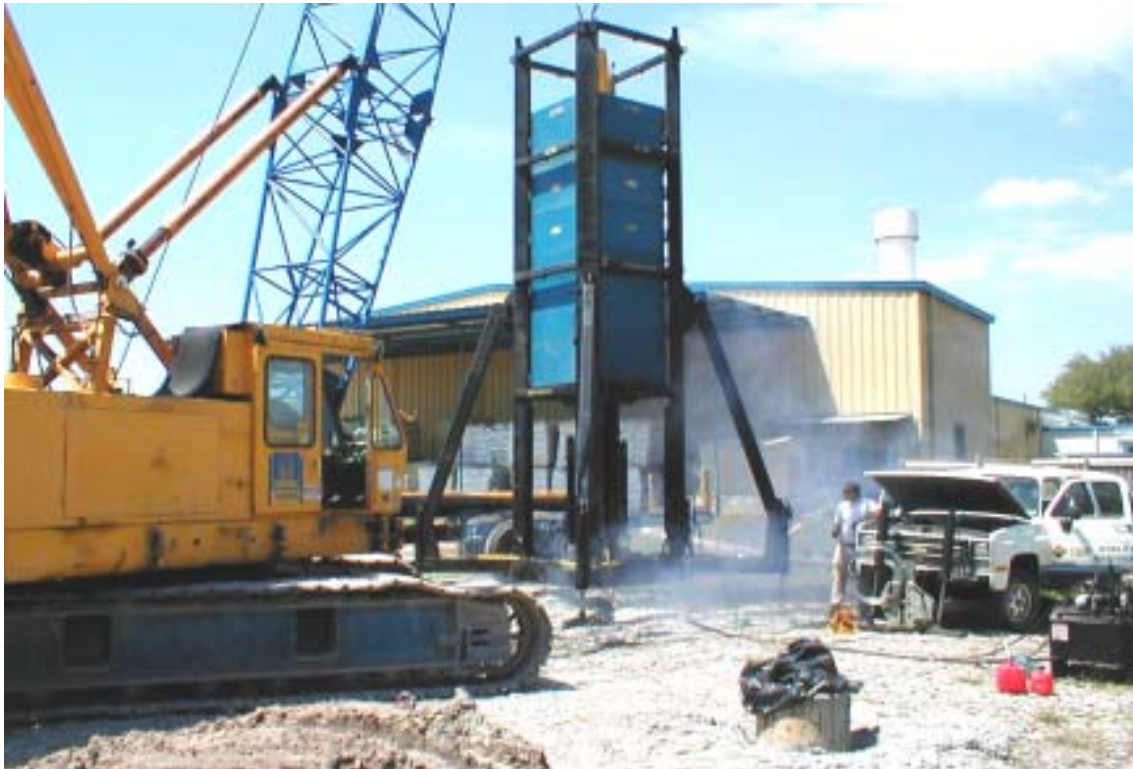
Figure 9. Static Load Test in Progress.
