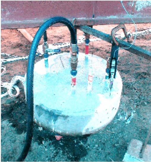
Fig. 4. Top of shaft receiving grout
