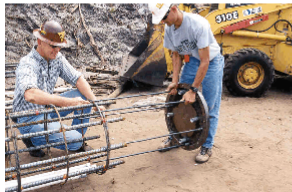
Fig. 3 Installation of grout distribution cell (Courtesy of Applied Foundation Testing, Inc.)
