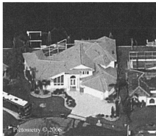
Fig. 7. Home with minor damage. 0.46–9.29 m 2 (5–100 ft 2 ) of missing tiles (Reprinted with permission, Pictometry International Corp. 2006).
