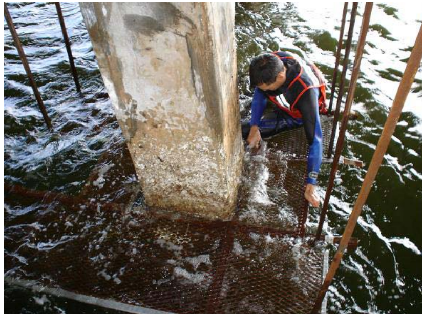
Figure 10 -- Scaffolding System, Gandy Bridge, Tampa
