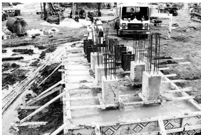
Fig. 8—Overview of cofferdam during concreting.
