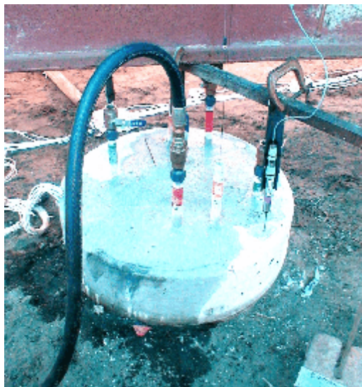
Fig. 4. Top of shaft receiving grout
