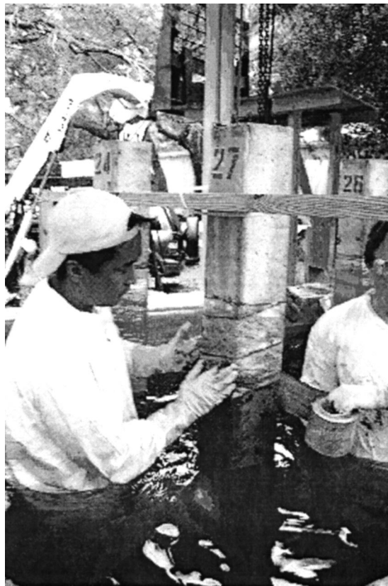
Fig. 1. Simulated underwater wrap
