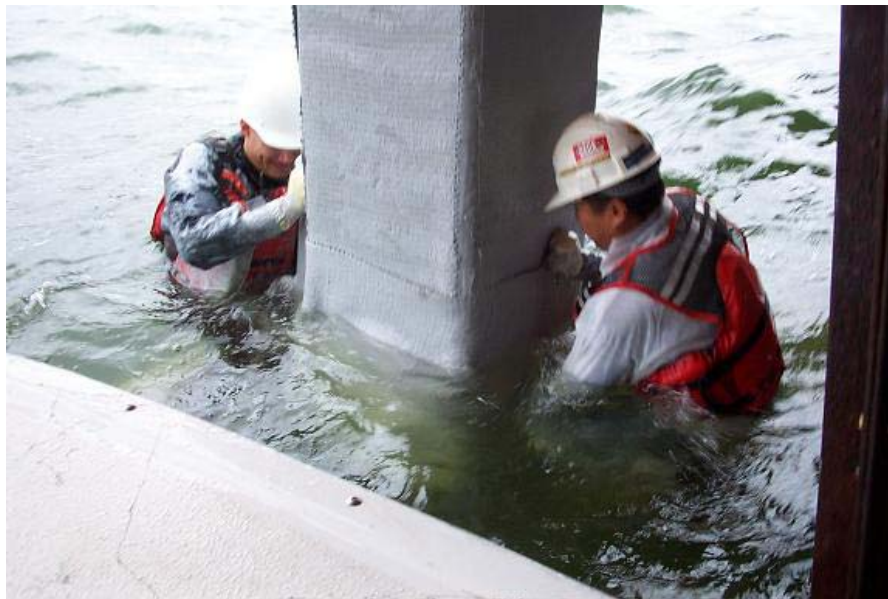
Figure 6 -- Underwater Wrapping, Friendship Trails Bridge, Tampa
