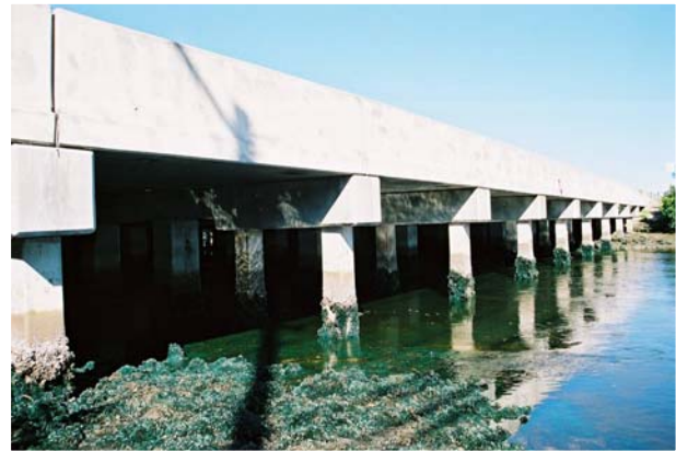
Figure – 1. Allen Creek Bridge piles
