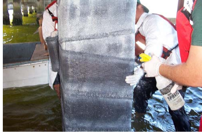
Figure 4. Applying transverse wrap
