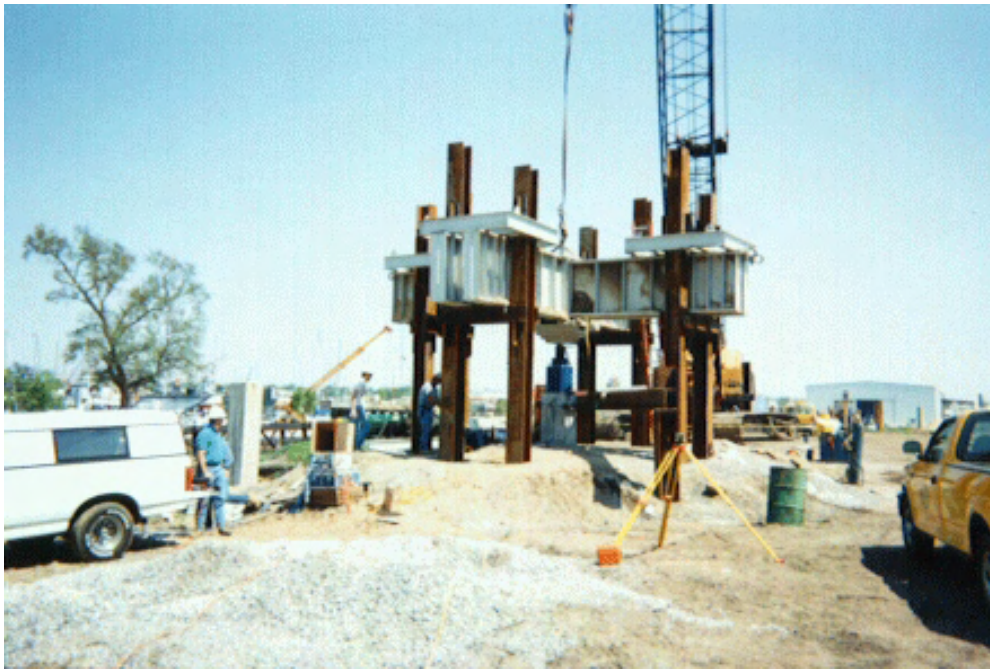
Figure 27 Static load test using 8, H-type reaction piles; 1200 ton.
