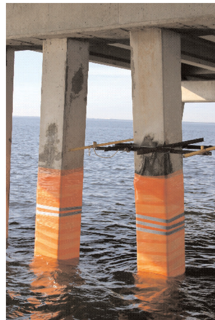
FIGURE 7 View of shrink-wrapped FRP repaired piles, Gandy Bridge, Tampa Bay.
