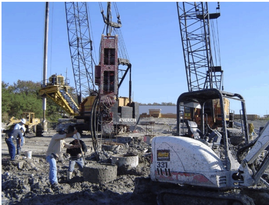
Figure 4 Shaft Construction at Port of Tampa
