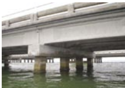
Fig. 2: The four piles of Bent 100 selected for FRP repair
