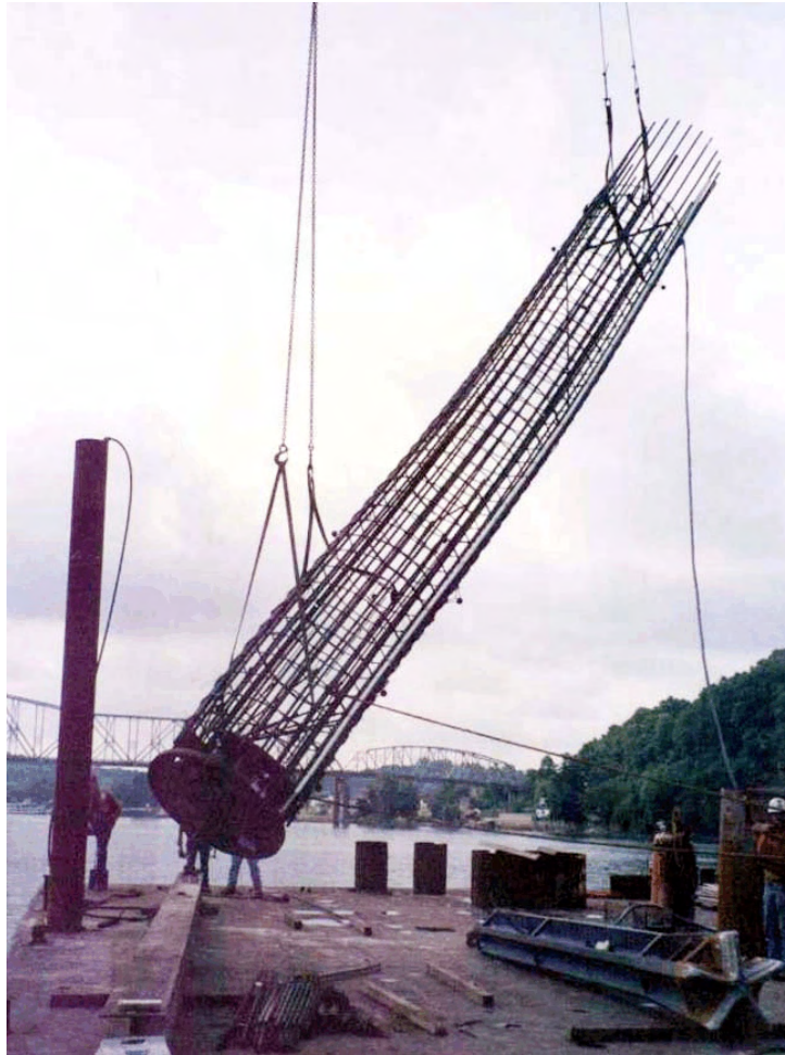
Figure 30 O Cell and cage lifted for installation (Courtesy of LoadTest, Inc.).
