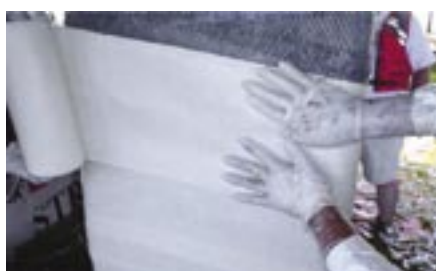
Fig. 8: Placement of glass fiber veil over bidirectional wrap
