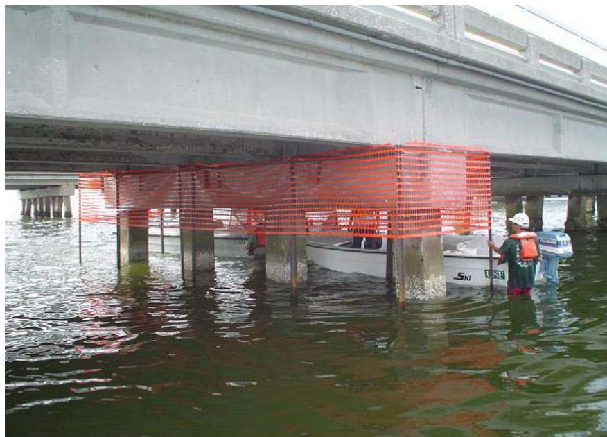
Figure 4 -- Scaffolding System, Friendship Trails Bridge, Tampa, FL
