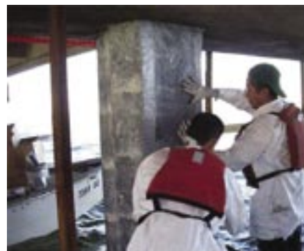
Fig. 6: Installation of unidirectional wrap on primed surface
