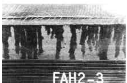
(c) Loose edge of CFRP.
