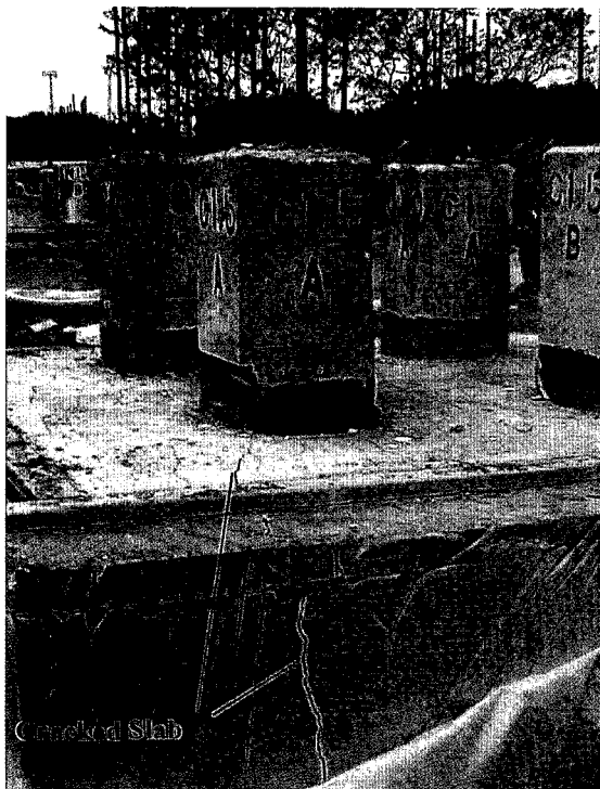
Figure 16: Seal Slab Cracks During Testing
