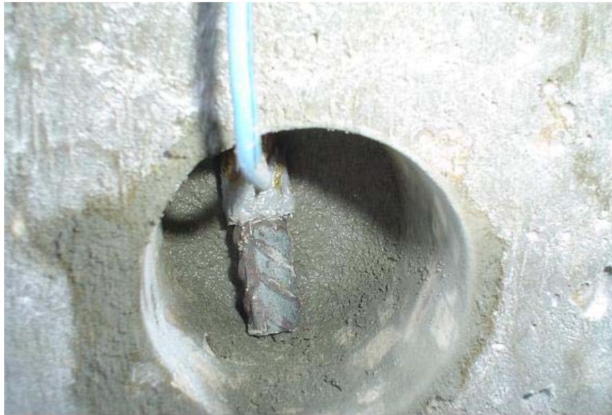
Figure 5 -- Rebar Probe Installation
