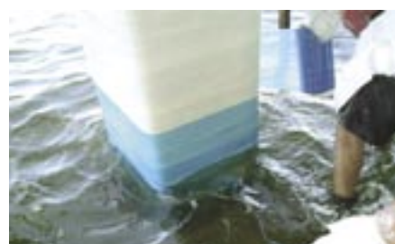
Fig. 9: Placement of plastic shrink-wrap over glass fiber veil
