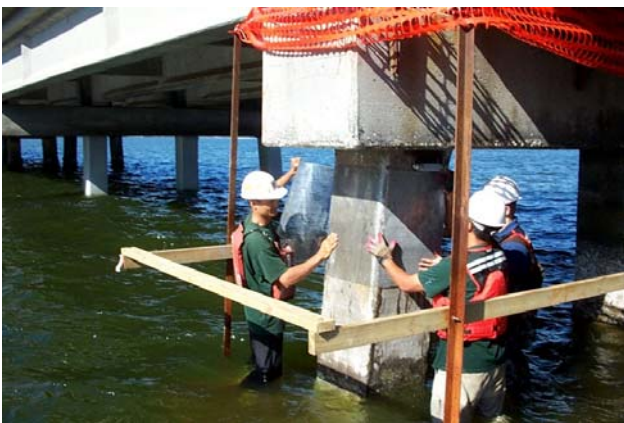
Figure – 4. Scaffold system for deep water access
