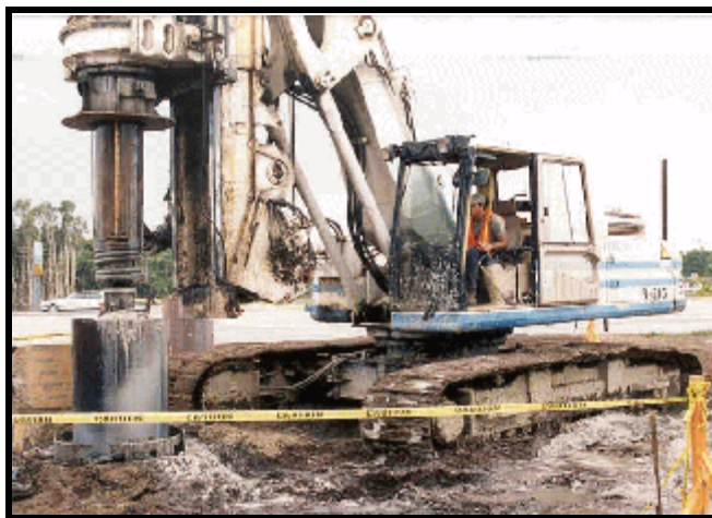
Figure 6. Test Shaft Installation.
