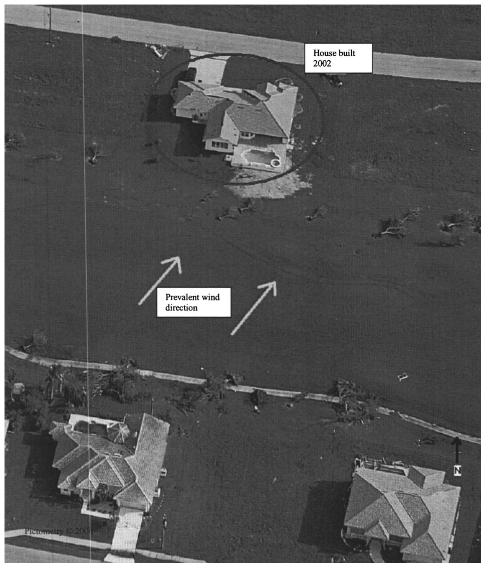
Fig. 16. Damage along ridges. Houses upwind show little damage (Reprinted with permission, Pictometry International Corp. 2006).
