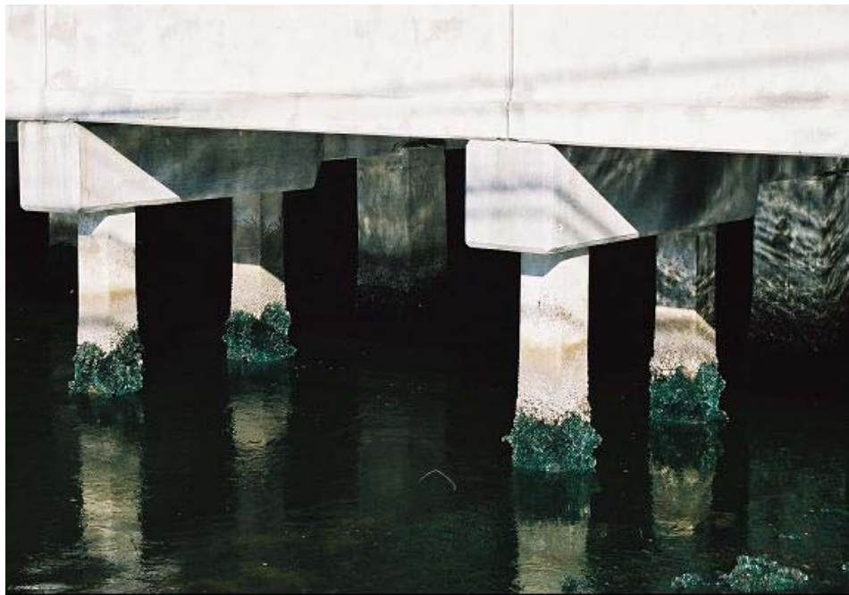
Figure 2 -- Marine Growth, Allen Creek Bridge, Clearwater
