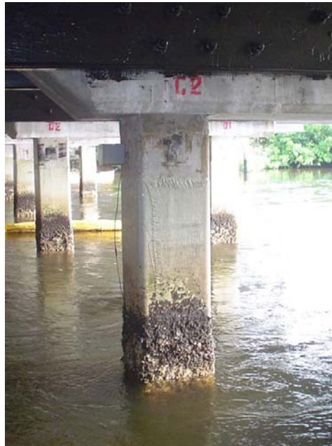
Figure 12 -- View of Wrapped Piles, Allen Creek Bridge, Clearwater after Two Years
