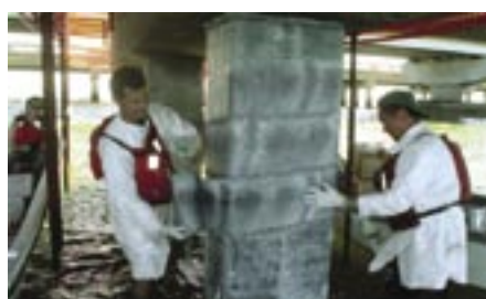
Fig. 7: Installation of bidirectional wrap to provide transverse reinforcement
