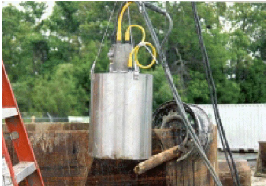
Figure 18 Miniature shaft inspection device (Courtesy of Applied Foundation Testing, Inc.)
