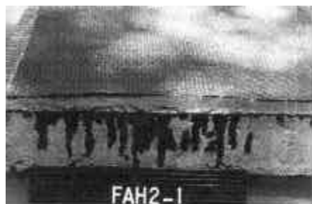
(a) Minor defects at edges of CFRP.
