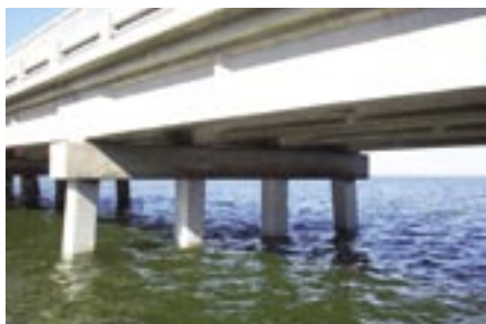
Fig. 10: Installation of UV-protective coating (plastic shrink-wrap removed)
