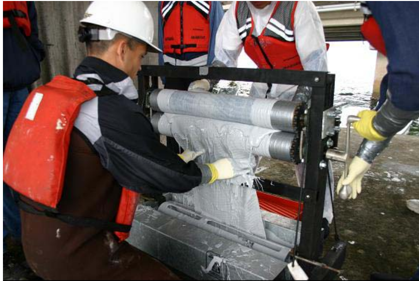
Figure 7 -- On-Site Saturation, Friendship Trails Bridge, Tampa
