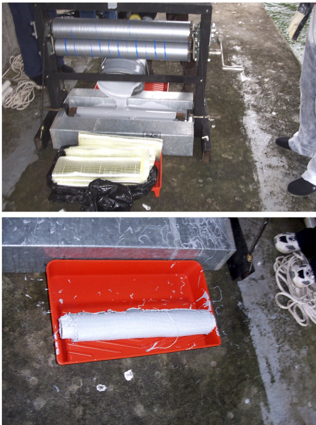
Fig. 8. On-site saturation of fiberglass fabric.
