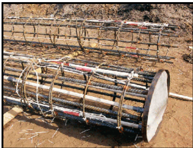
Figure 5. Instrumented test shaft cages.
