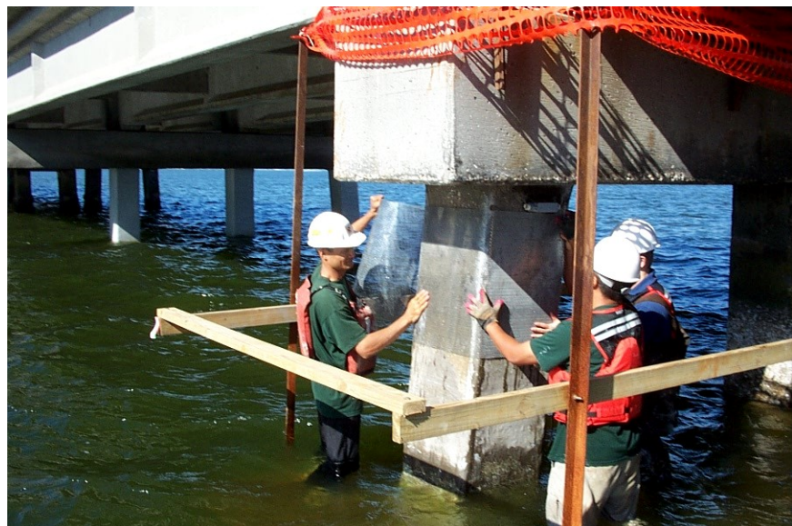
Figure 2. Scaffolding used for repair
