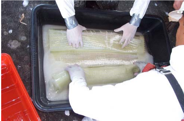
Figure 3. Saturating FRP on site
