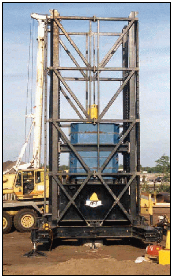
Figure 10. 2000 ton Statnamic load test.
