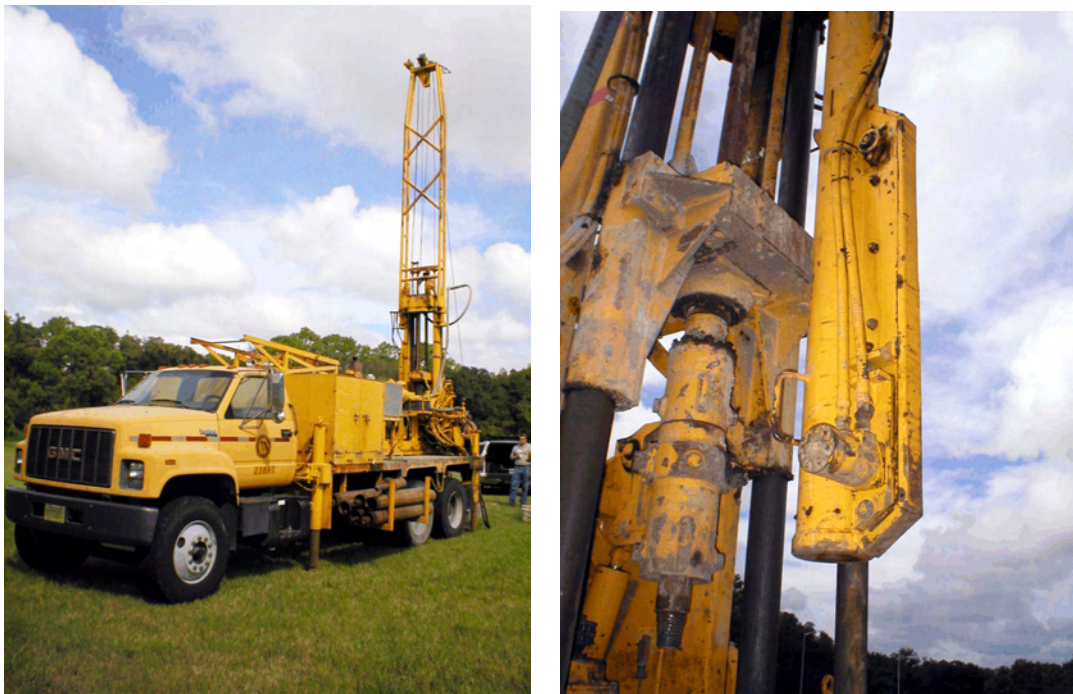
Figure 6 Truck-mount drill rig (left), chain driven automatic SPT hammer (right).
