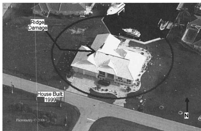
Fig. 18. Damage due to wind along ridges (Reprinted with permission, Pictometry International Corp. 2006)
