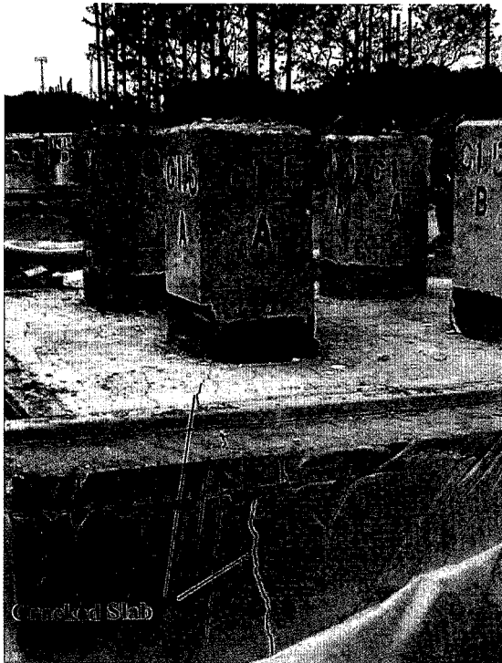
Figure 16: Seal Slab Cracks During Testing
