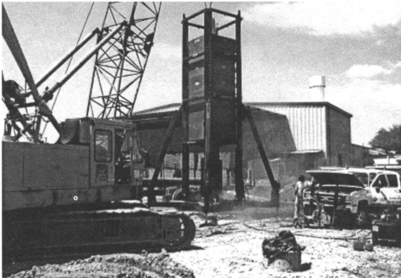
Figure 9. Statnamic Load Test in Progress.
