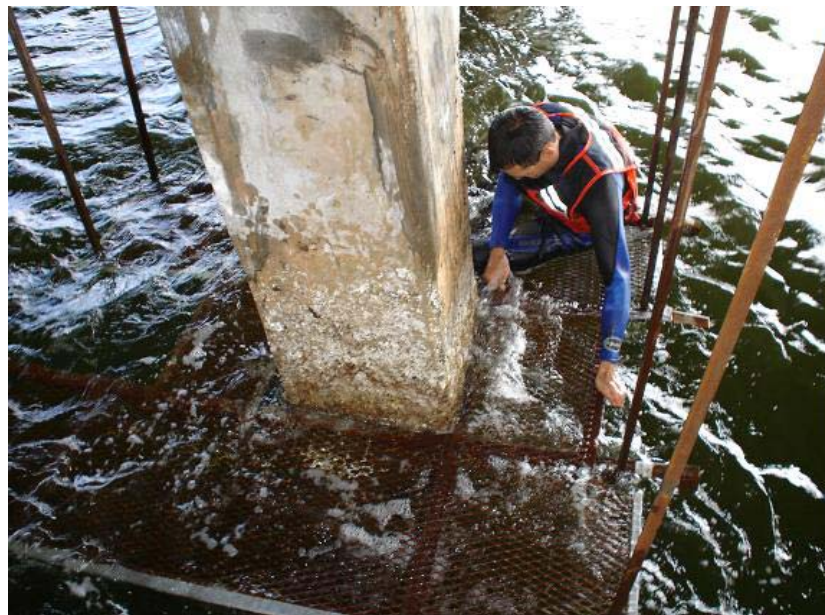
Figure 10 -- Scaffolding System, Gandy Bridge, Tampa
