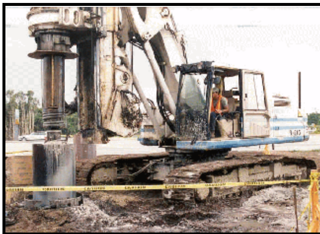
Figure 6. Test Shaft Installation.
