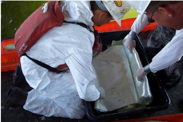
Fig. 5. Saturating FRP on site
