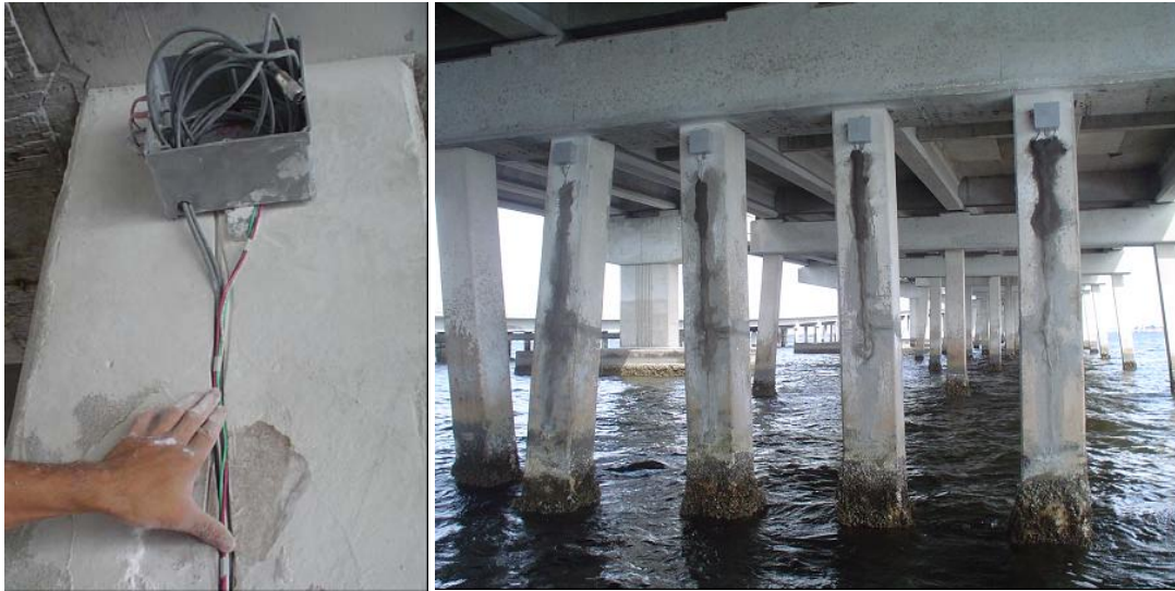
Figure 8 – Installing junction box and wiring.
