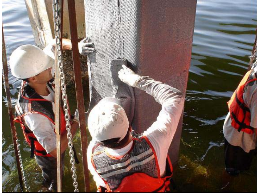
Figure 11 -- Underwater Wrapping, Gandy Bridge, Tampa
