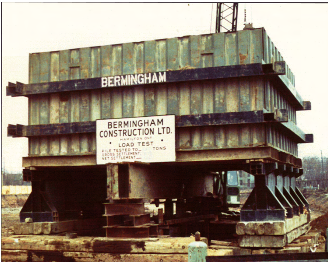
Figure 26 Kentledge load test setup; 400 ton (Courtesy of Bermingham Construction, Ltd).
