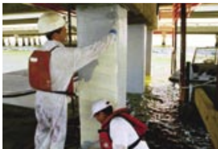
Fig. 10: Installation of UV-protective coating (plastic shrink-wrap removed)
