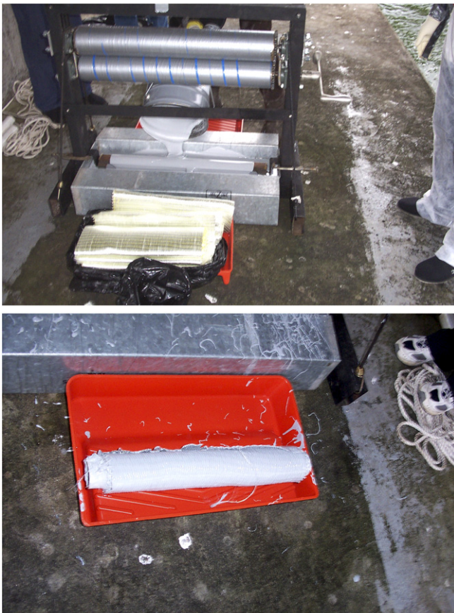
Fig. 8. On-site saturation of fiberglass fabric.
