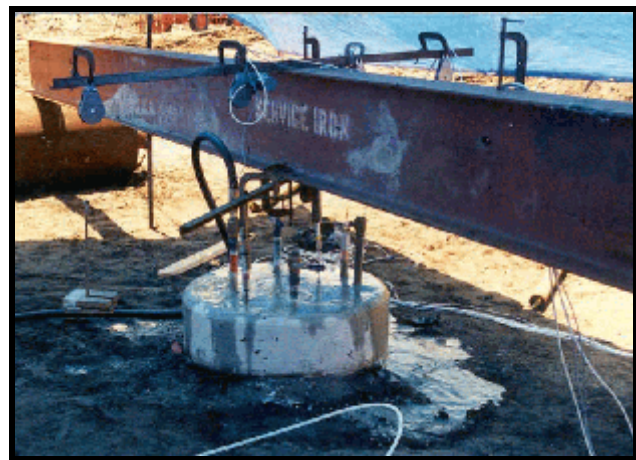
Figure 9. Monitoring test shaft during grouting.
