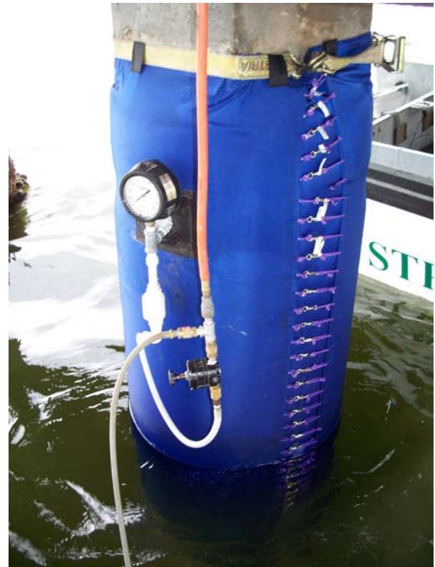
Figure - 6. Pressure bag securing FRP while curing
