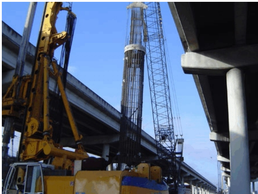
Figure 5 Drilled Shaft Construction at the Crosstown Expressway
