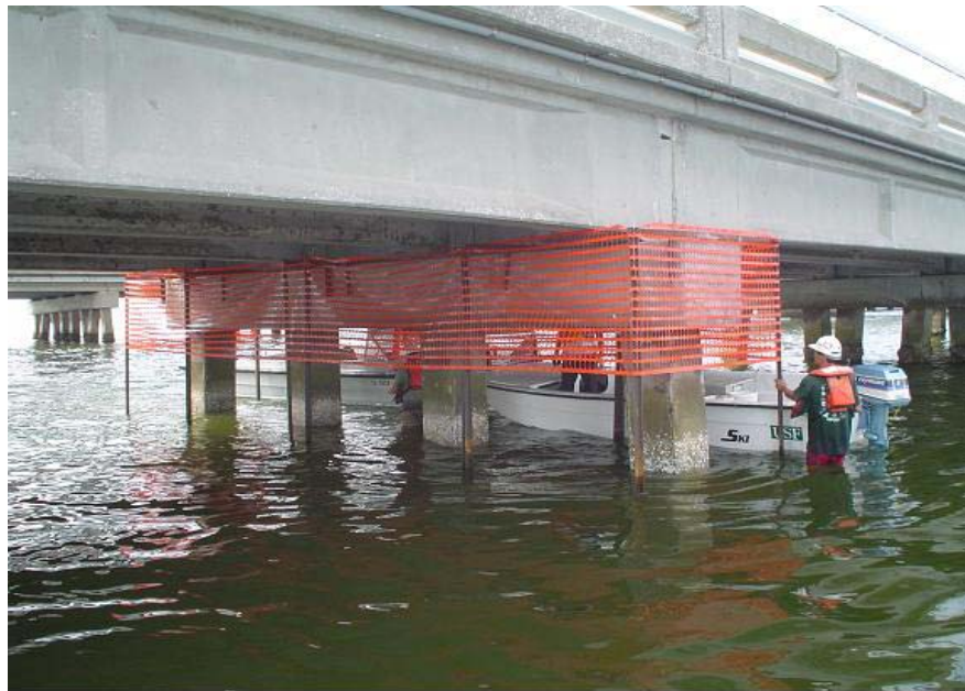
Figure 4 -- Scaffolding System, Friendship Trails Bridge, Tampa, FL
