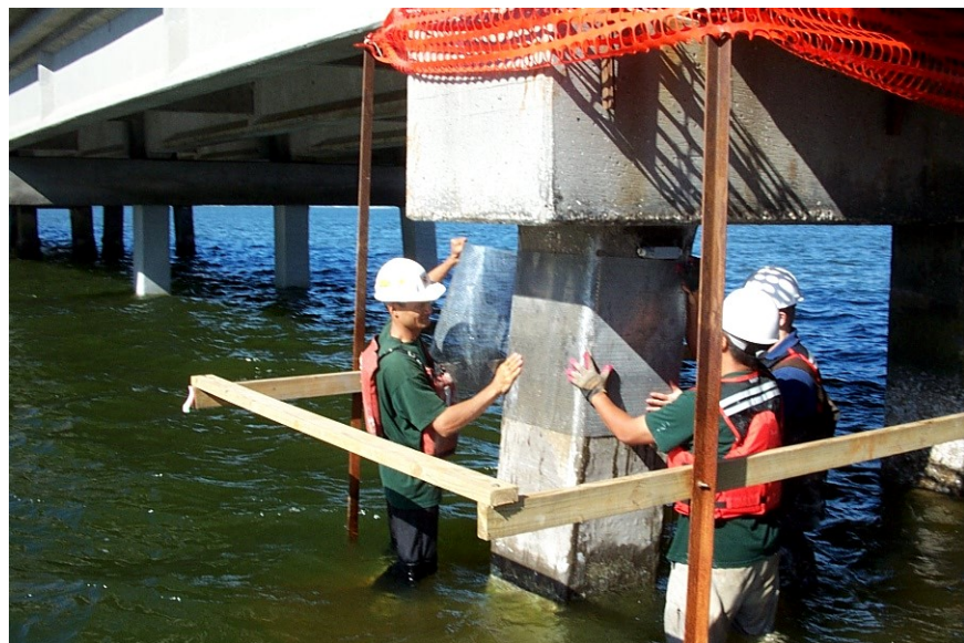
Figure 2. Scaffolding used for repair
