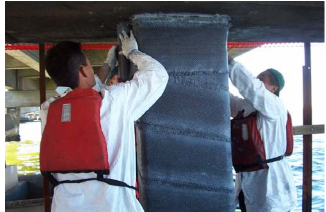
Fig. 6. Applying transverse wrap
