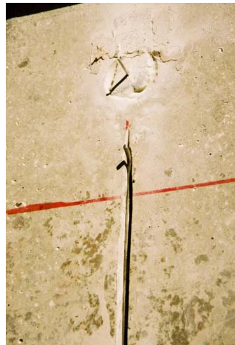
Figure – 2. Embedded stainless steel electrode
