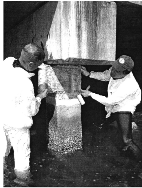
Fig. 18. Wrapping witness panel for bond test
