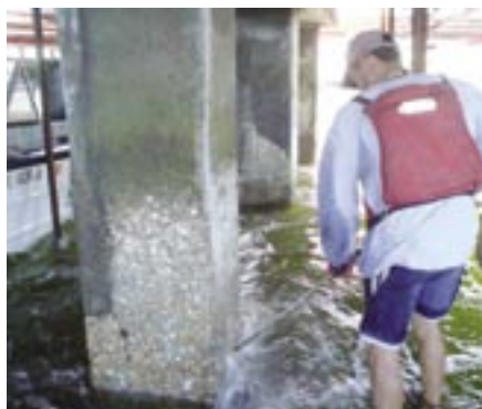
Fig. 5: Pressure-washing of repair zone using fresh water
