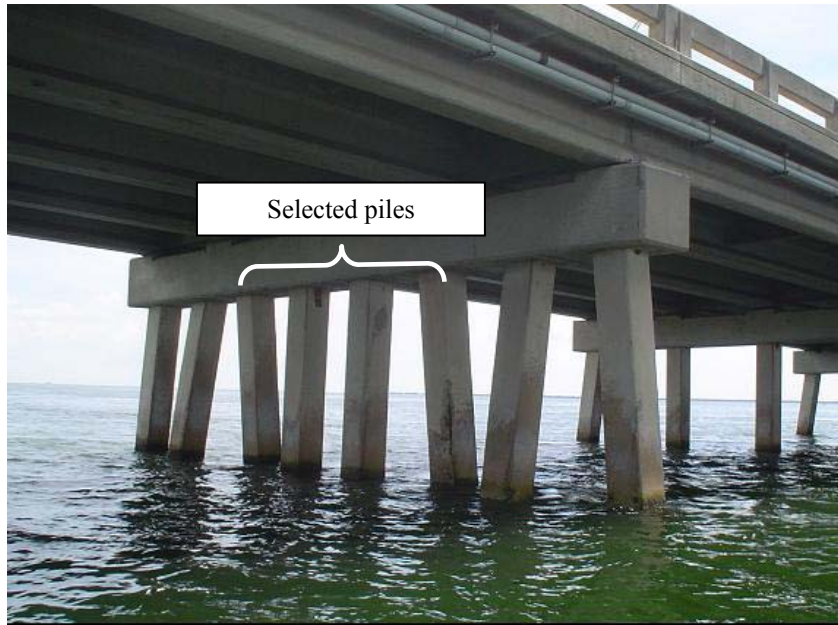
Figure 9 -- Selected Piles, Gandy Bridge, Tampa
