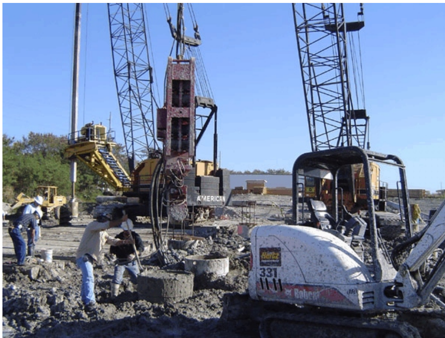
Figure 4 Shaft Construction at Port of Tampa
