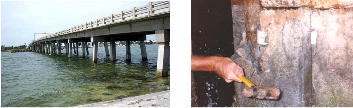
Figure 1. Jacketed pile repair (left) and view with jacket removed (right)
