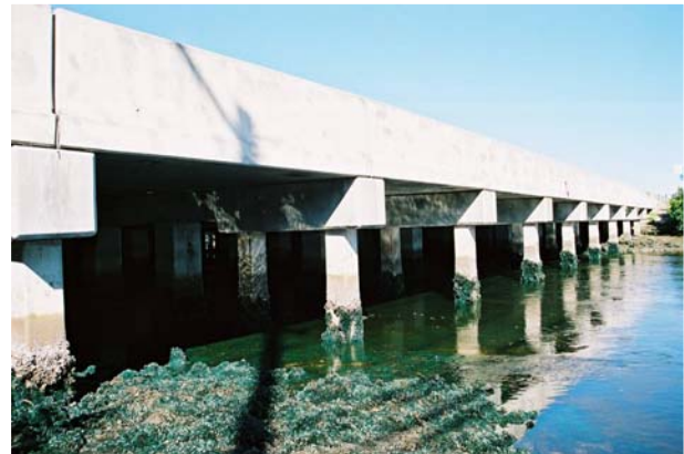
Figure – 1. Allen Creek Bridge piles
