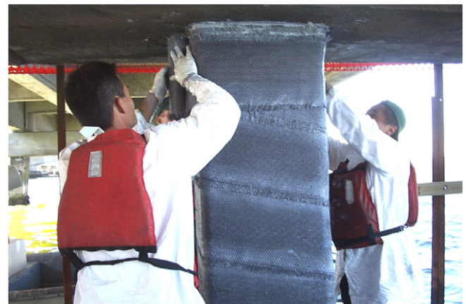
Fig. 7. Applying second transverse CFRP layer.
