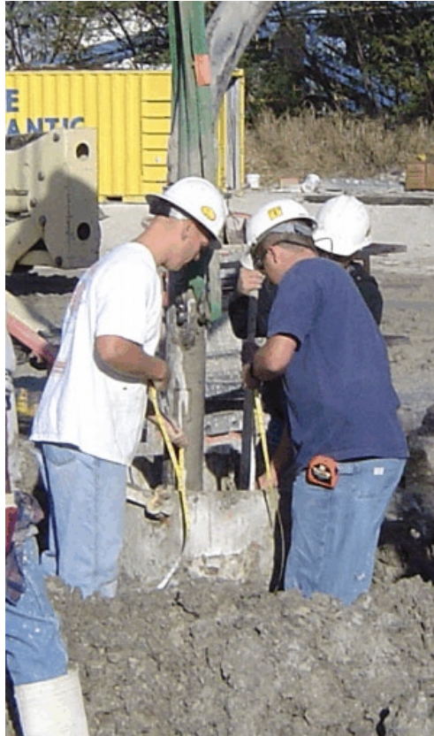
Figure 3 Rising Concrete Level Measured Inside and Outside Reinforcing Cage
