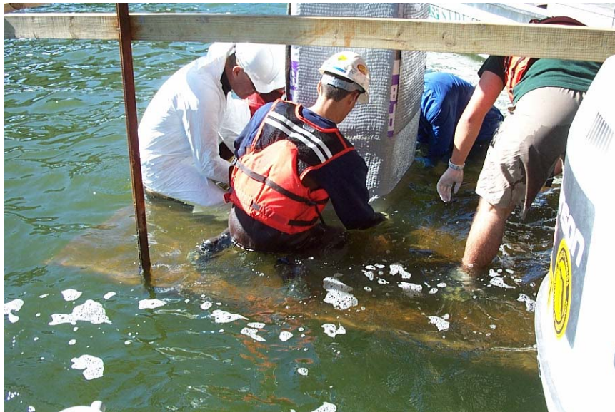
Fig. 4. Scaffolding used for repair
