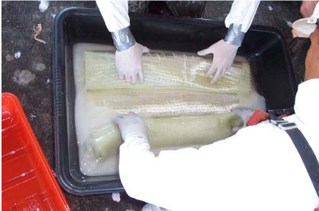
Figure 3. Saturating FRP on site
