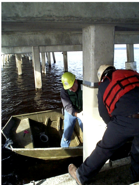
Fig. 4. Underwater repair using a boat and divers (Courtesy: Air Logistics).
