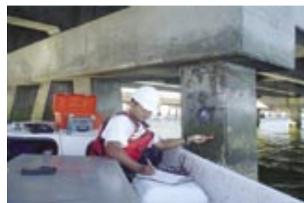
Fig. 3: Corrosion assessment using surface potential measurements per ASTM C 876 prior to repair
