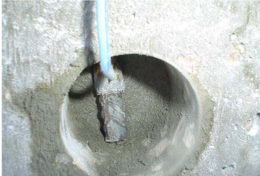
Figure 5 -- Rebar Probe Installation
