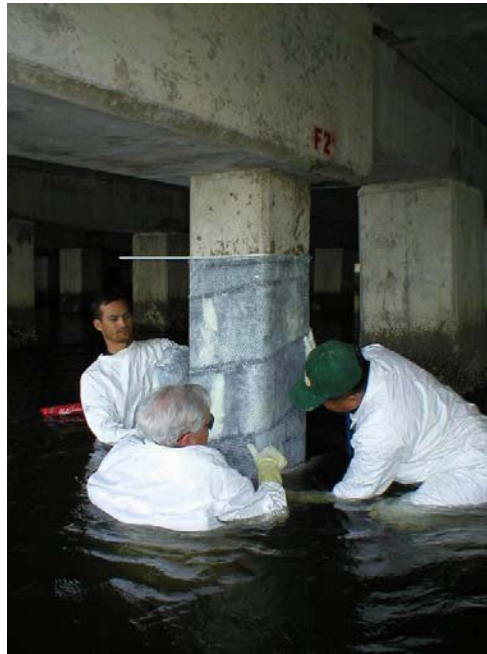
Figure 3 -- Underwater Wrapping, Allen Creek Bridge, Clearwater
