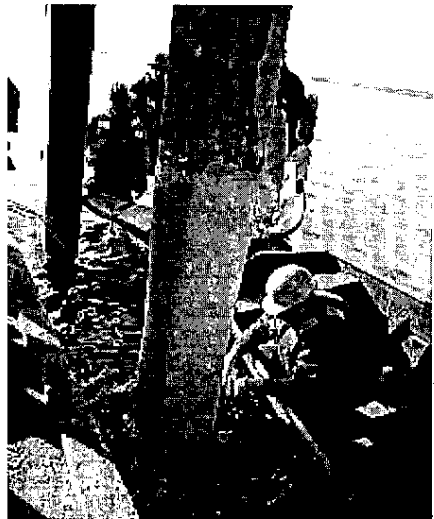
Fig.4 Underwater Wrap (courtesy Air Logistics, CA)
