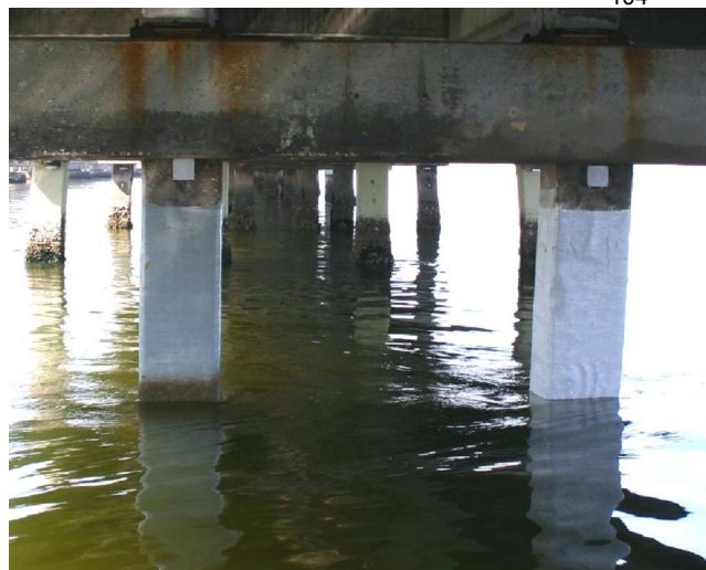
Fig. 15. Piles after FRP repair with UV coating
