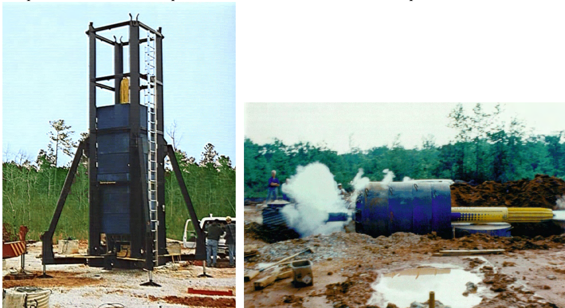
Figure 32 Axial statnamic test setup (left), lateral statnamic test in progress (right).
