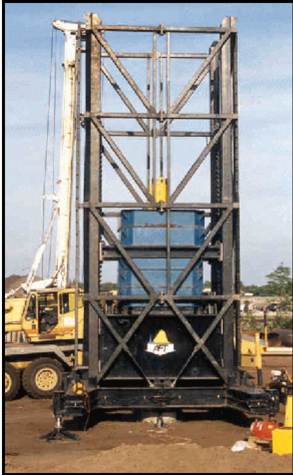
Figure 10. 2000 ton Statnamic load test.
