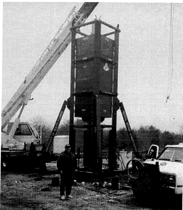
Figure 3. View of Statnamic load test apparatus over test pile #2
