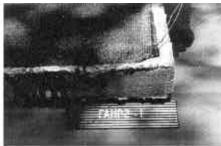
(b) Frayed corner from poor top coat.
