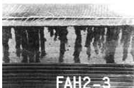
(c) Loose edge of CFRP.
