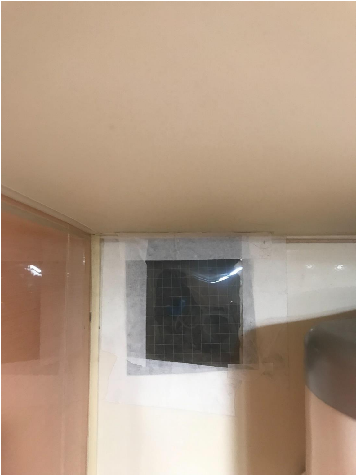
Figure 4. Sealed vent in the bathroom of a residential apartment in Tomsk.
